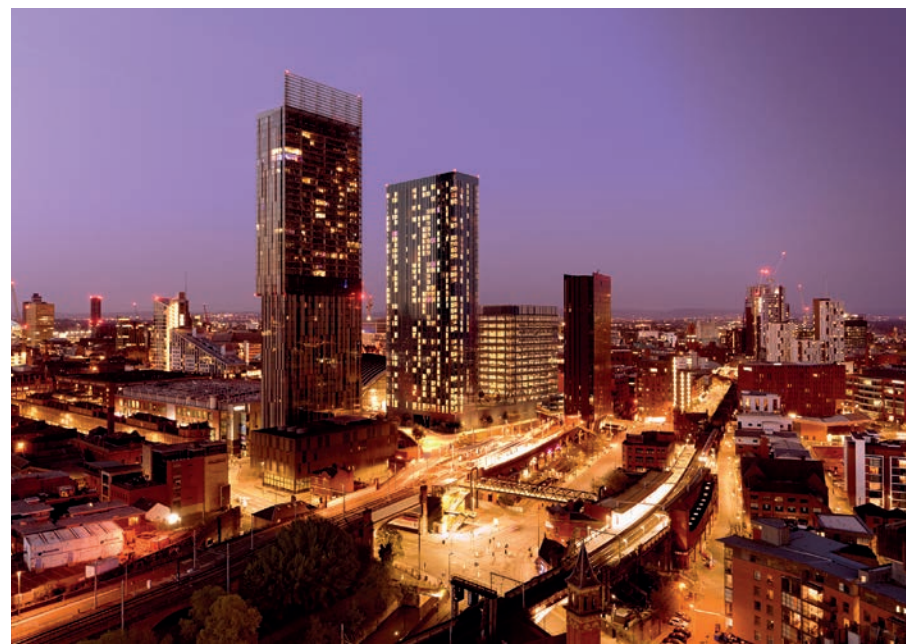
VIADUX GREAT BRIDGEWATER ST.
